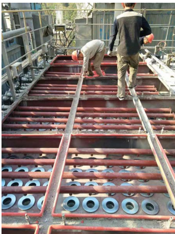
Installing the pleated bags on site.
