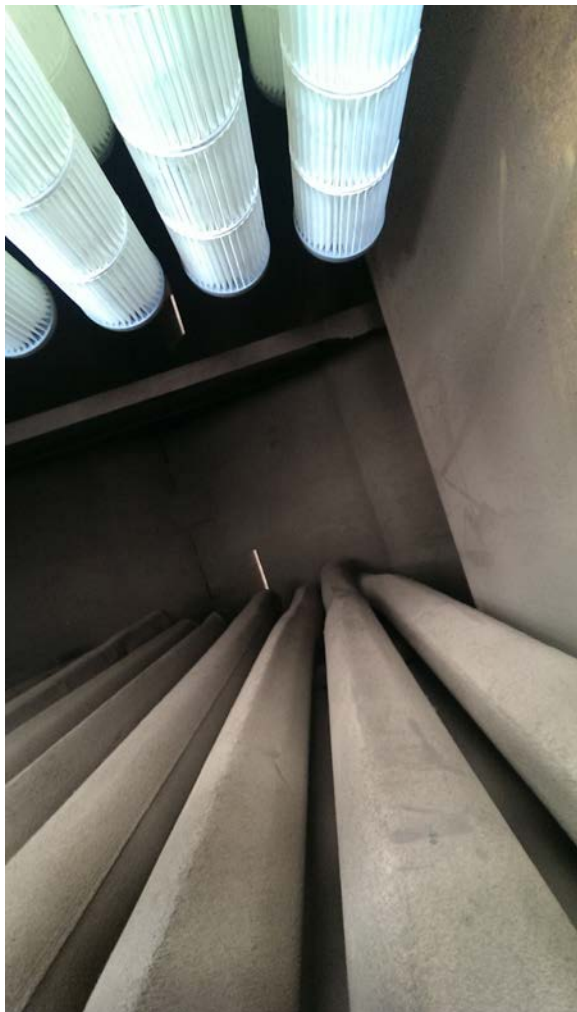
The difference in length between the pleated bags and filter bags.
